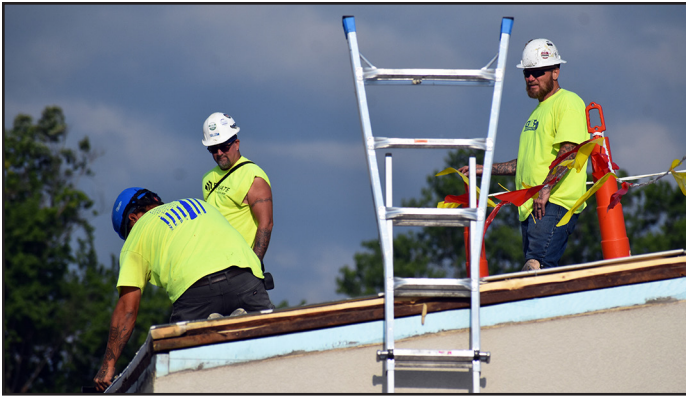
Workers are at Pardeeville Middle School replacing the roof during the month of July, a project that will finish in the middle of August.
